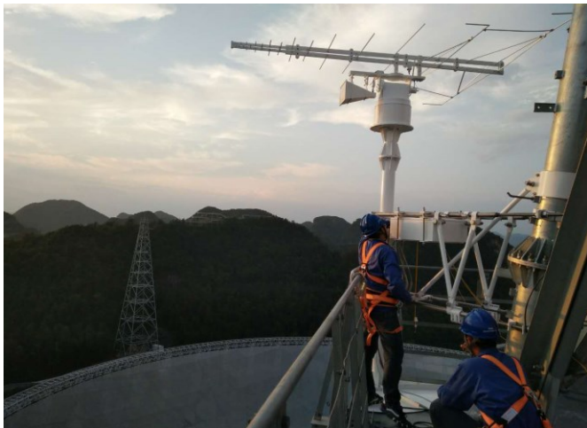
RFI monitoring antenna in FAST site
