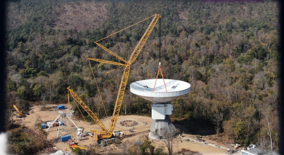
Current status of structure building (Aug 2020)
