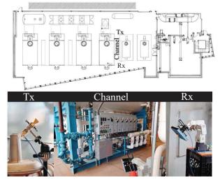
Figure 2: Small utility plant (a) floor plan and (b) measurement set-up.
